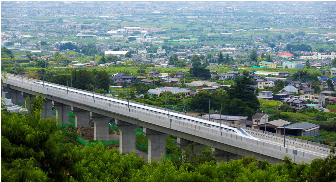
Figure 6: Picture of Yamanashi Maglev Line Viaduct Section (example from Japan)
